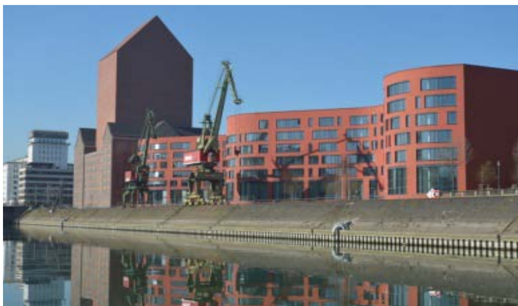
“Photo of the year” : the new premises of the State Archives of North Rhine-Westphalia in Duisburg (two cranes in front of the building belong to the historical ensemble), photo: the State Archives, Mr. Peter Fröhlich.
